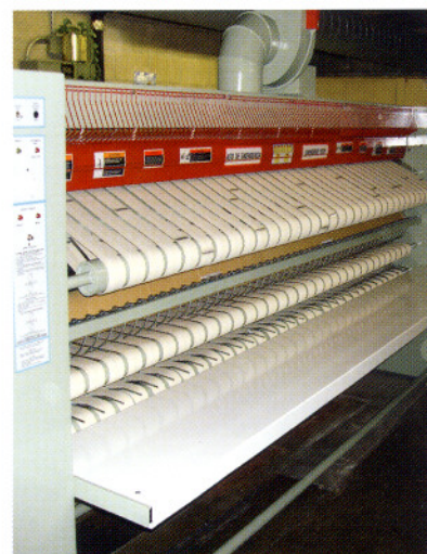
New Installation at "The Orlando"
